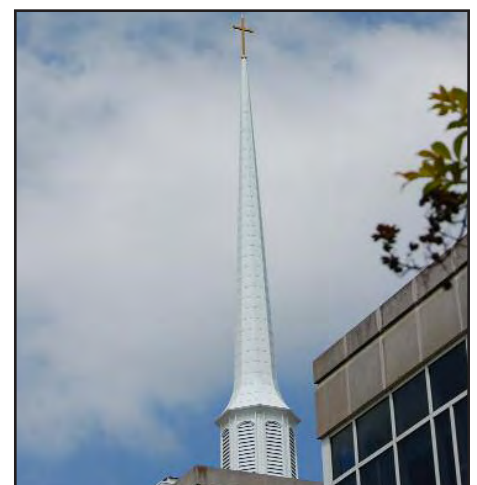
The new steeple in place.
