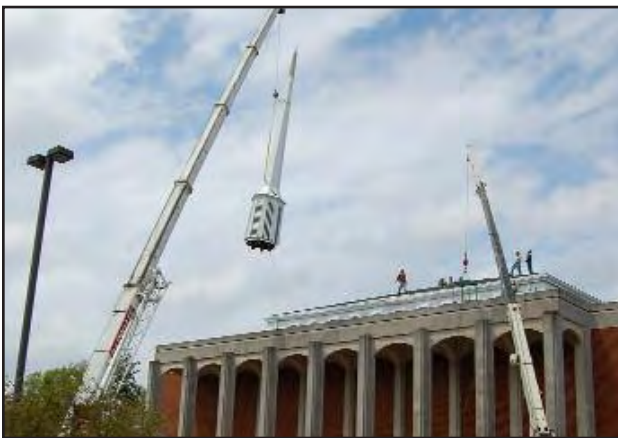
The old steeple being lifted off the sanctuary roof.
